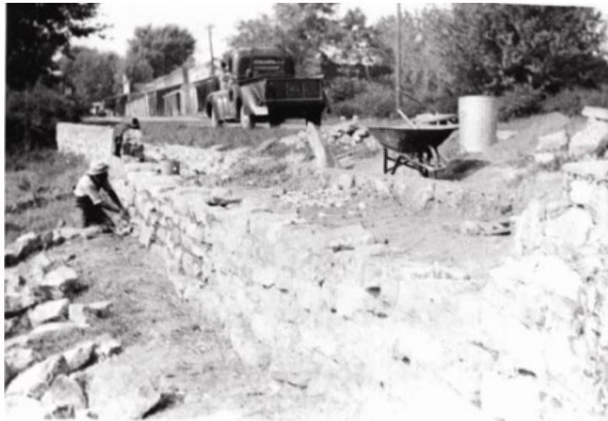
Civilian Conservation Corps workers constructing a retaining wall at Arrow Rock State Historic Site in the 1930s.
